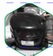
Works on single Compressor.
